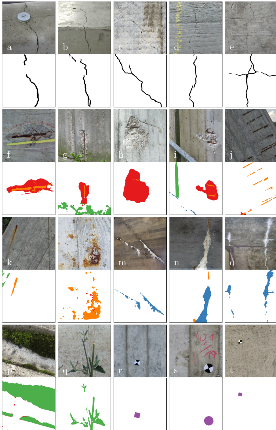
Fig. 3: Qualitative results of HMA on the test set. Classes: crack (black), spalling (red), corrosion (orange), efflorescence (blue), vegetation (green), and control point (purple).
